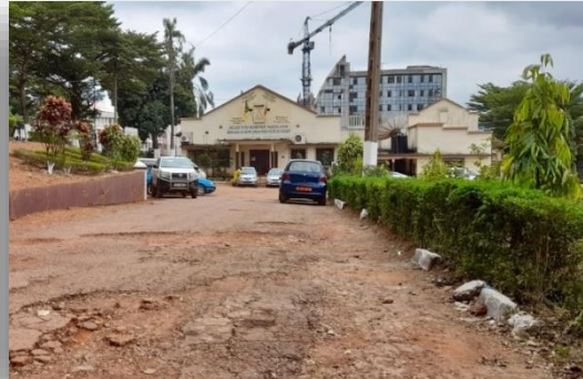
Photo 01: ARCAM building, the current Yaoundé Linguistic Pilot Centre. Photo Tele Djosseu 2024
